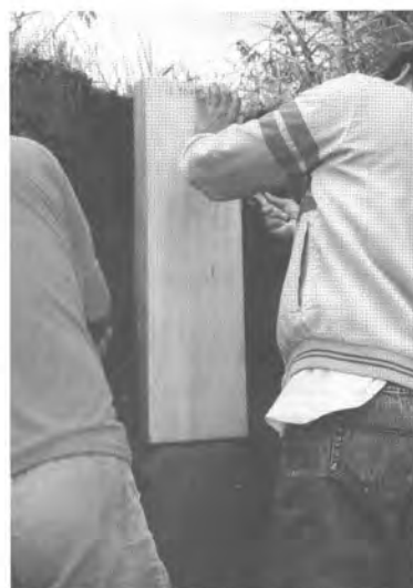
Photo 5. The soil materials behind the box are removed.
