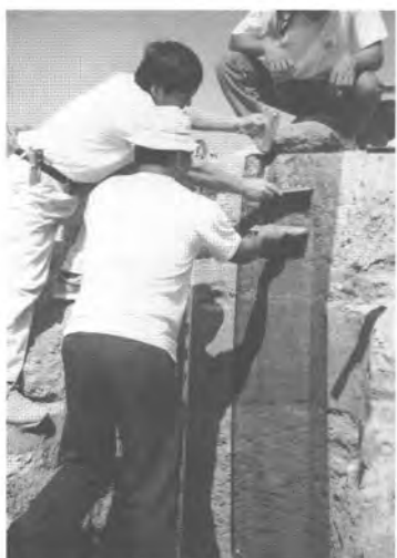
Photo 18. The Tomack NS-10 resin is applied on the cloth.
