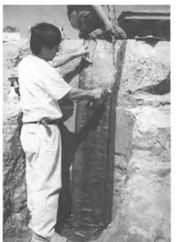
Photo19. Enough water is sprayed for hardening.
