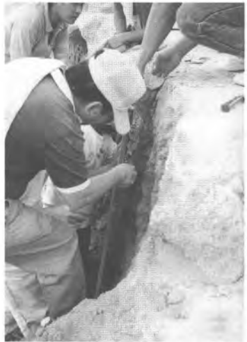
Photo 22. The soil materials behind the soil column are removed.
