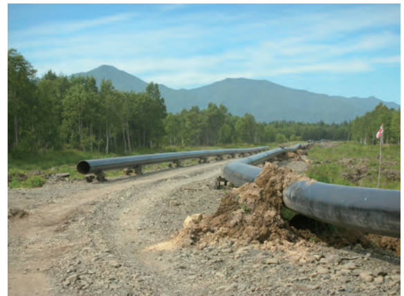
Photo 6. Pipe line under construction.
