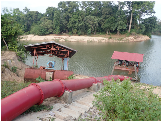
Photo 23. An irrigation facility that pumps water from a pond in the Panomsai village
