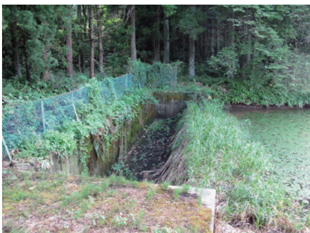
Fig.2-5 洪水吐流入口付近に繁茂する雑草 The weed which grows thick in front of spillway
