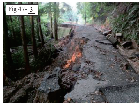
Fig. 50 堤体下流道路の崩落 Collapsed road of downstream bank
