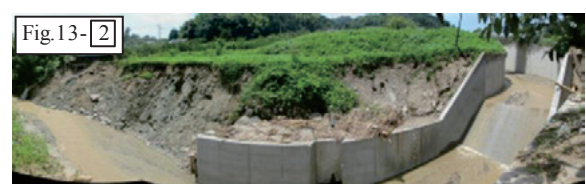
Fig. 15 梅ヶ谷 1 ため池の堤体と洪水吐水路 Bank and spillway channel at Umegatani 1 pond
