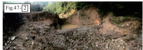
Fig. 49 洪水吐および堤体の崩落 Failure of spillway and bank
