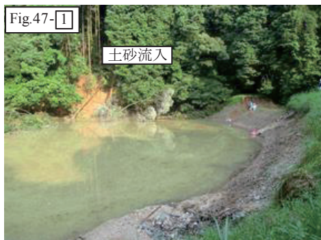
Fig. 48 ムクロジため池の堆砂状況 Sand and mud flowed into Mukuroji pond
