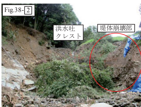
Fig. 40 洪水吐水路の崩落 Failure of spillway channel
