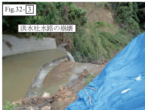
Fig. 35 洪水吐水路の崩落 Failure of spillway channel
