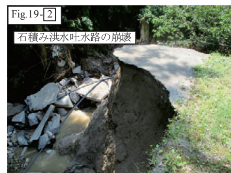
Fig. 21 生津ため池の洪水吐水路 Spillway channel at Namazu pond
