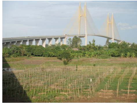
Photo 2. Neak Loeung Bridge between Kandal Province and Prey Veng Province across the Mekong River.
