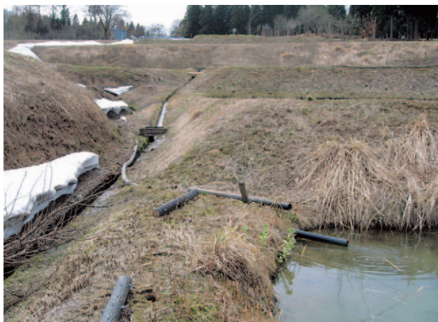
Fig. 110 Water intake system from streams to cultivated paddies.
