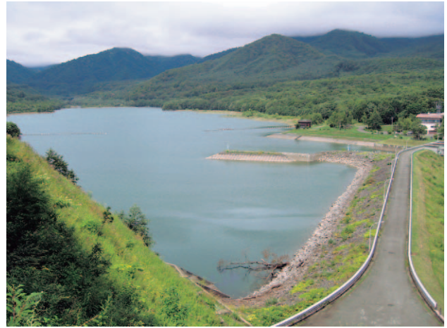
Fig. 7 Photograph of Sasagamine dam looking west. See Fig. 5 for its location.
