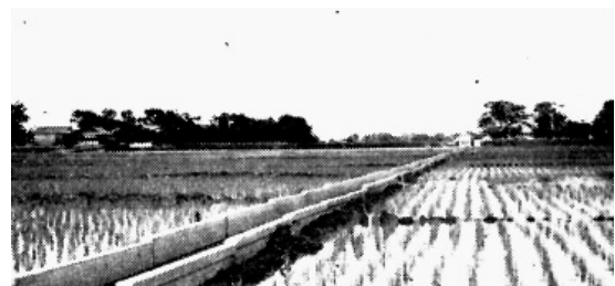
Fig.2-19 躯体の浮上りによるずれ(土木学会, 1966) Damage of canal joint due to uplift of canal body
