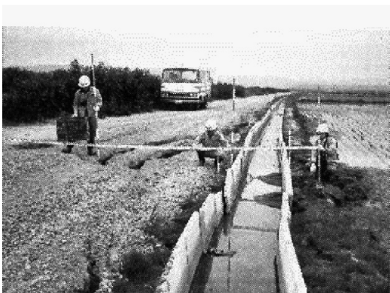
Fig.2-23 不同沈下による躯体のずれ (土木学会, 1986) Shift of canal body due to differential settlement
