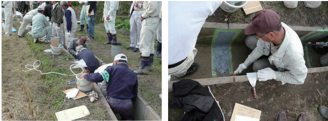
Fig.5-26 目地補修の研修状況 Training for farmers to repair canal joint
