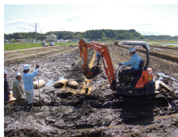
Fig. 6 暗渠排水整備 Subsurface drainage improvement
