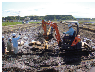
Fig. 13 暗渠排水の施工状況 Installation of subsurface drainage
