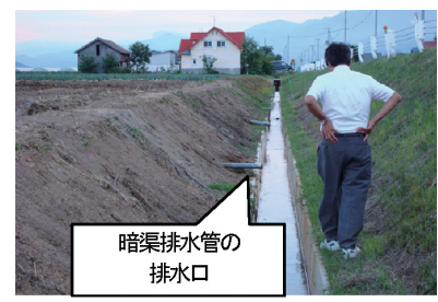
Fig. 7 排水路整備 Drainage channel improvement
