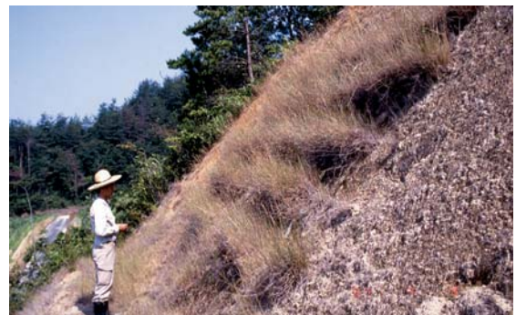
Fig.30 肥料袋に沿ってベルト状に生育したレドトップ Redtop which grew in belt shape along fertilizer bags
