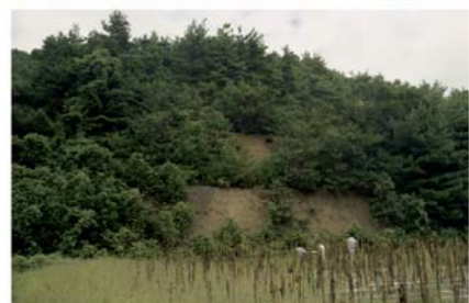
Fig.28 肥料袋工追肥試験区設定法面の变化 Change of the slope of topdressing by fertilizer bags
