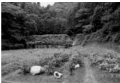
Photo 3-1 迫の益ため池の決壊状況（下流側より望む） Breached Sakonoeki dam (viewed from downstream)
