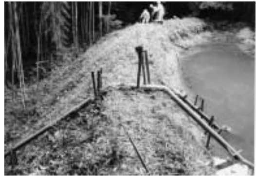
Photo 5-4 仏光寺ため池の堤体 Embankment of Bukkouji dam
