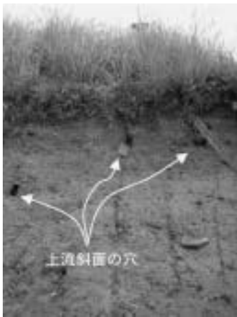
Photo 3-12 山崎ため池の上流斜面の穴 Hall on upstream slope of Yamazaki dam
