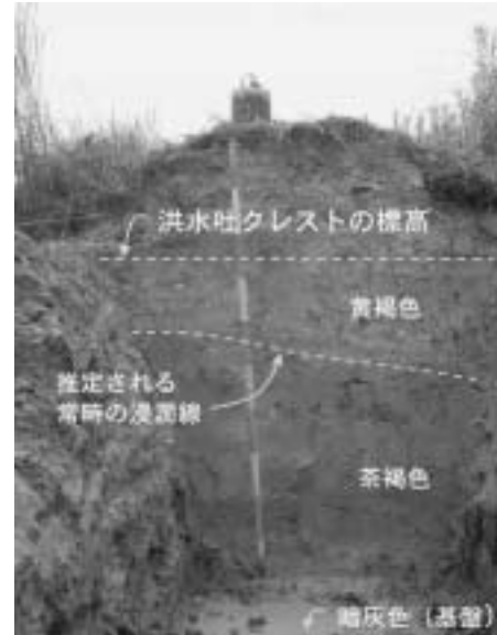
Photo 3-8 堤体掘削面の観察 Cross section of embankment
