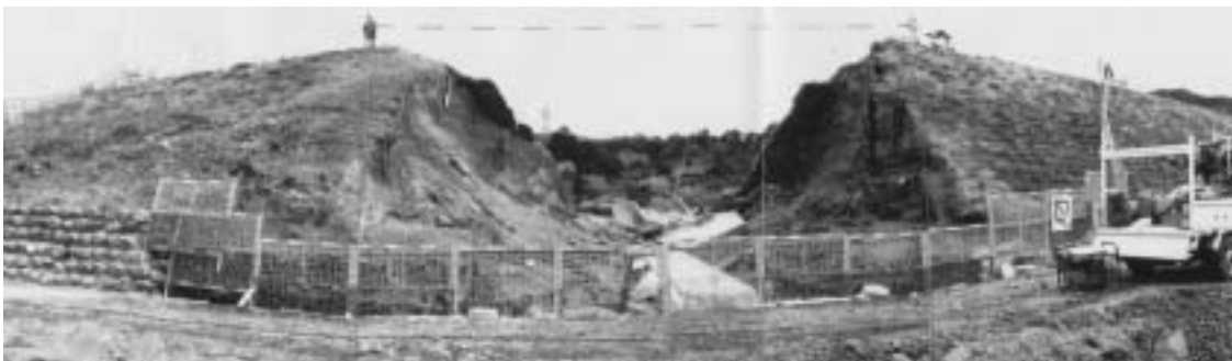
Photo 3-22 内原野ため池の決壊状況 (下流より) Condition of breach of Uchiharano dam (viewed from downstream)
