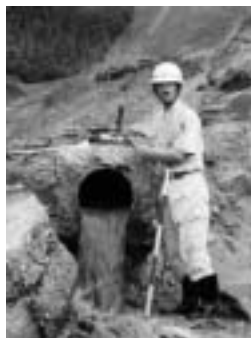
Photo 3-20 麻生ため池の底樋 Outlet pipe of Asou dam
