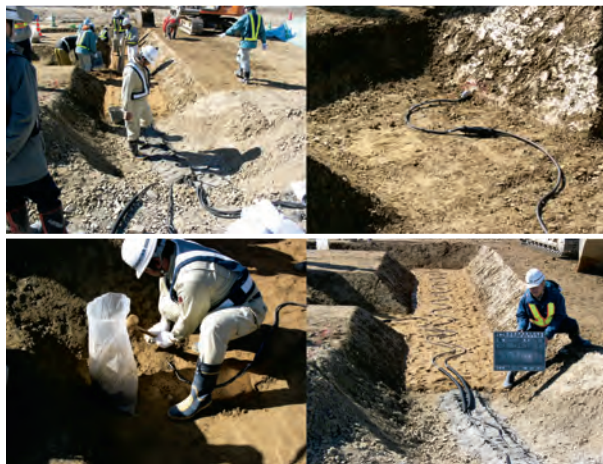
Fig.5 ケーブル式間隙水圧計の設置状況 Views of setting up the transducers with cable
