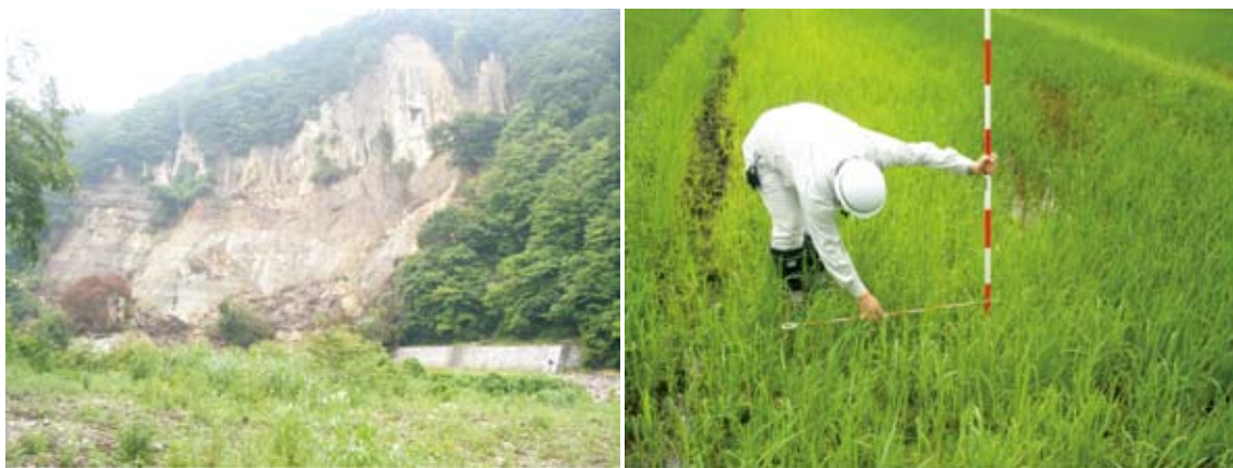
Fig.18 下り松用水の斜面崩落状況（左）水田の地盤沈下（右、楓木立地区） The slope collapse on the Sagarimatsu channel (left), a subsidence in a paddy field at Hanokidate district (right)
