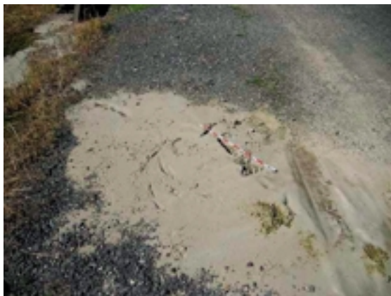
Fig.18 道路での噴砂の跡 Sand boil on a road surface
