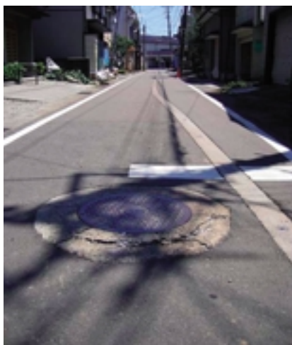
Fig.8 改良土で埋戻された区間の地表面 Undamaged road surface where improved soil was used
