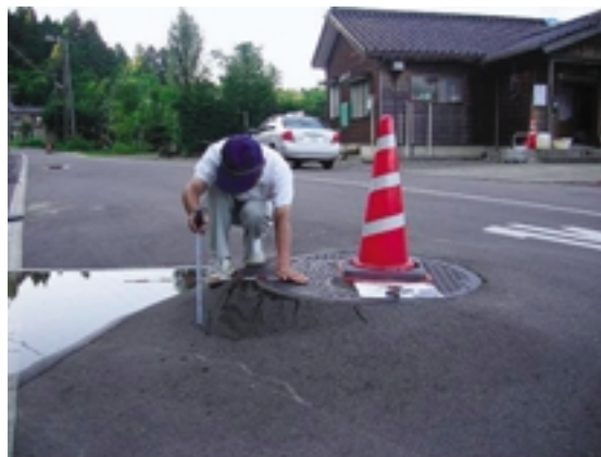
Fig.20 マンホール周辺の路面沈下 Settlement of road surface near a manhole
