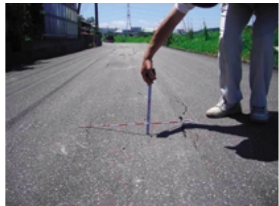
Fig.6 管路の埋戻し部分の路面沈下 Settlement of road surface
