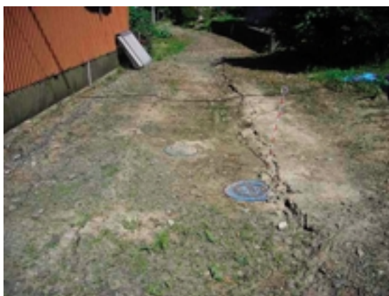
Fig.15 管路埋戻し部分の地表面沈下 Settlement of ground surface
