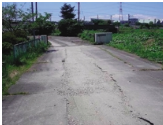
Fig.10 沈下した路面部分に敷均された碎石 Crushed stone used as fill after settlement of road surface.
