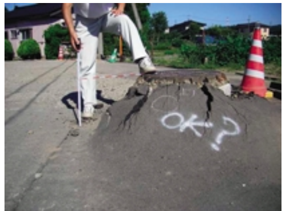
Fig.16 マンホールの浮上 Uplift of a manhole
