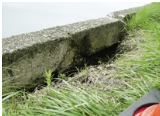
Fig.40 護岸壁の破損（坂田池） Damage to a revetment wall
