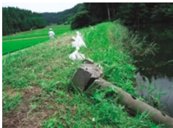
Fig.15 斜樋の損傷 Damage to inlet works
