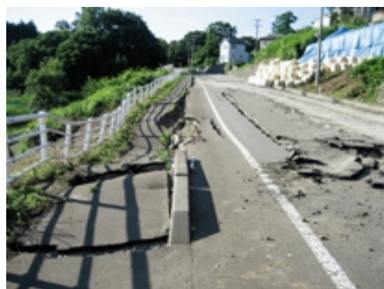
Fig.48 左岸側管理用道路の被害(桐の木谷池) Damage to an abutment of a management road
