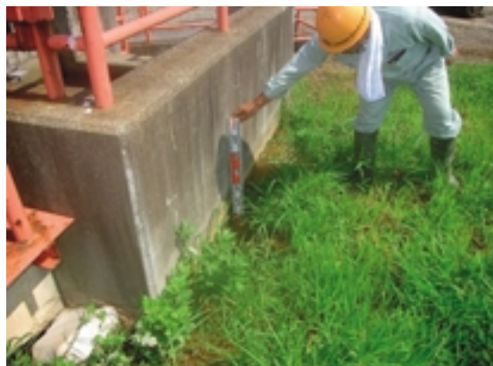
Fig.22 第2取水口の沈下, 変形 (大池) Settlement of foundation at outlet works
