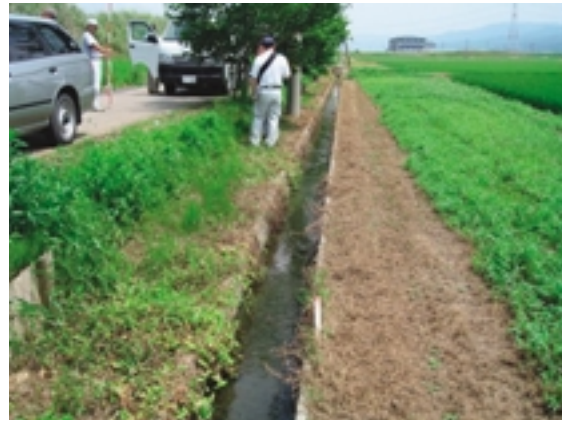
Fig. 59 幹線水路の変状 Deformation of main canal
