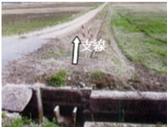
Fig. 55 支線水路U字溝の分水枘への貫入 (石川県提供資料) Penetration of a concrete flume into a distribution tank
