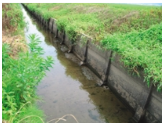
Fig. 38 周辺地盤の沈下に伴う水路の不陸 Deformation of canal base caused by ground settlement
