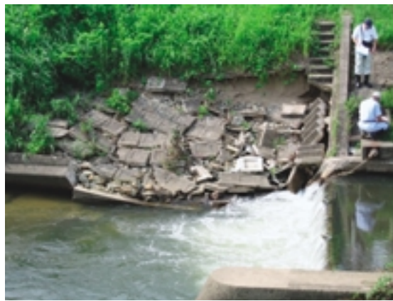
Fig. 17 頭首工護岸工の被災状況（調査時） Damages to protection work at the time of investigation
