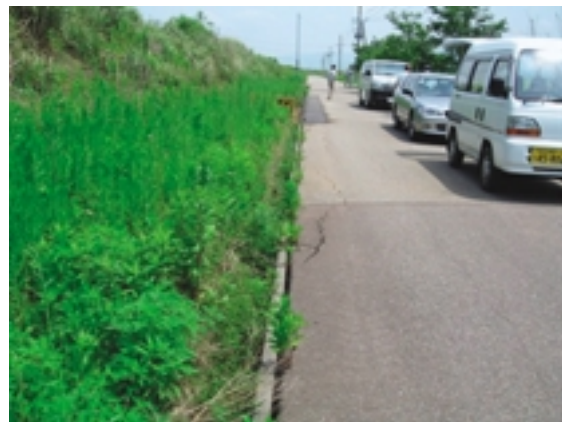
Fig. 60 邑知漏干拓堤防法尻部の道路側溝の変状 Deformation of a channel at the toe of a bank in Otagata
