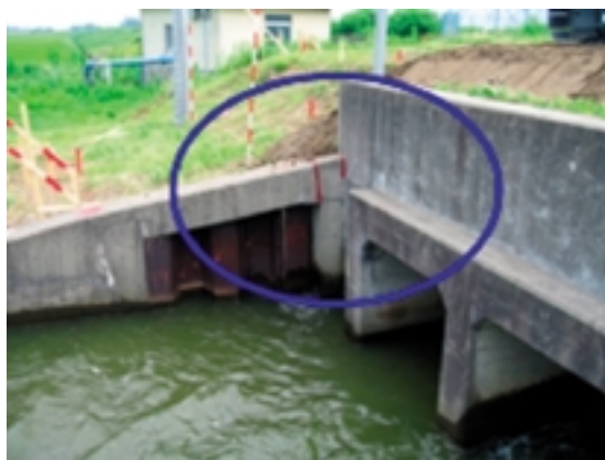
Fig. 50 排水樋門と矢板護岸工取り付け部からの漏水 Leakage from a joint between a sluice gate and sheet-pile
