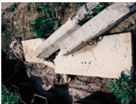
Fig. 25 柵板の破損状況 A damaged concrete panel
