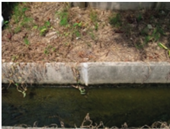
Fig. 58 幹線水路 U 字溝目地の修復状況 Repair of an opened joint between concrete flumes
