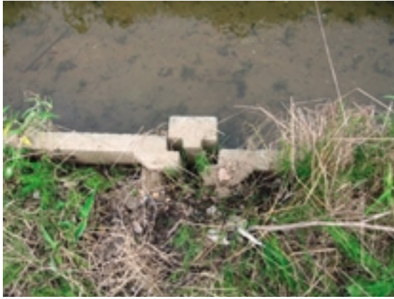
Fig. 39 柵工枠と柵板のずれ Gap between frame and panels
