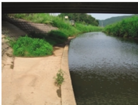
Fig. 11 頭首工直上流部（右岸）の河川護岸工の前傾 Inclination of covering work at the head work
