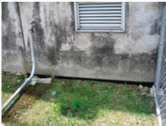
Fig. 53 建屋と地面との隙間 Opening between a building and the ground
