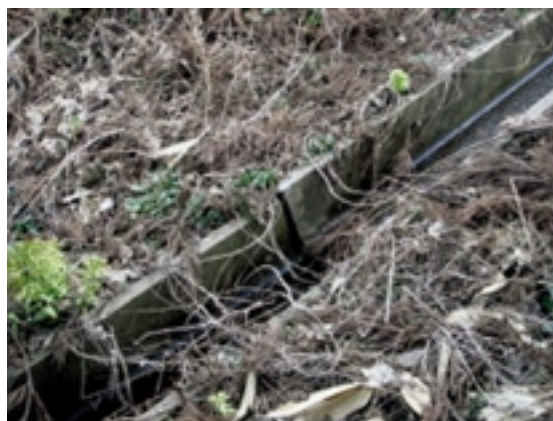
Fig.7 水路の目地の開き Opened joint of a drainage canal
