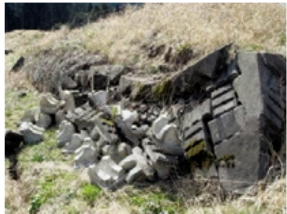
Fig.20 擁壁の崩壊 Close-up of retaining wall failure
