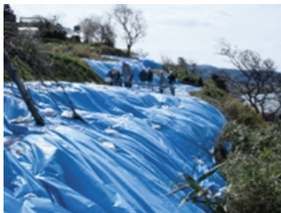
Fig.3 (a) 稲舟地区クラック箇所応急対応状況 Emergency countermeasures at a crack site in the Inafune area
