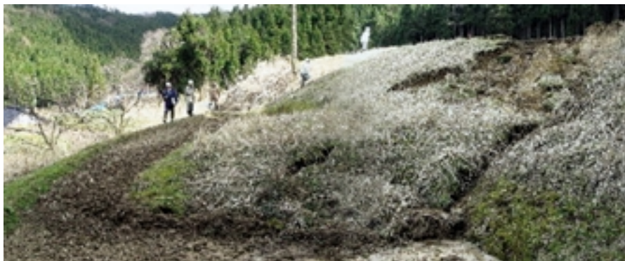
Fig.13 畦畔法面に生じた地すべり性崩壊 Landslide on a levee slope
