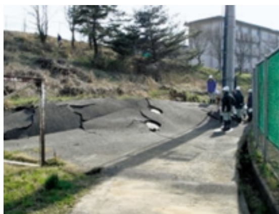
(b) 輪島実業高校地すべり末端隆起部 Upheaval in the toe area of the landslide at the Wajima Business High School
