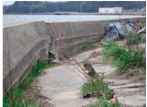
Fig.21 護岸工の移動と背面地盤の流失 Lateral movement of seawall and washout of back fill sand
