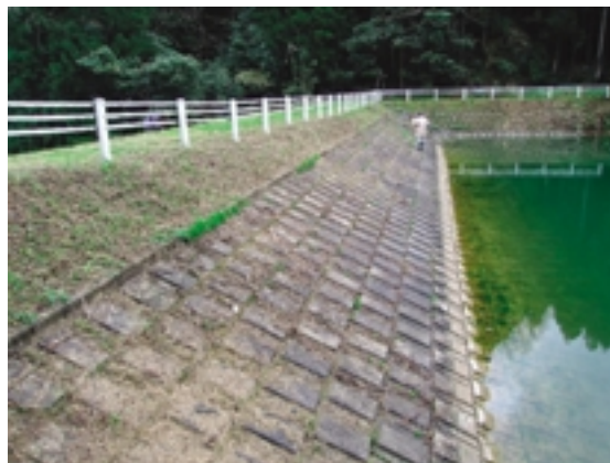
Fig.12 上流法面保護ブロックの沈下 Settlement of the concrete block mat on the upstream slope
