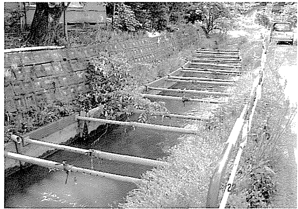
Photo 23 切梁による応急復旧 Urgent repair of canals with sturts
