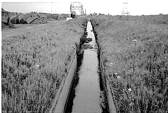
Photo 15 排水路の復旧状況 Restoration of drainage canals
