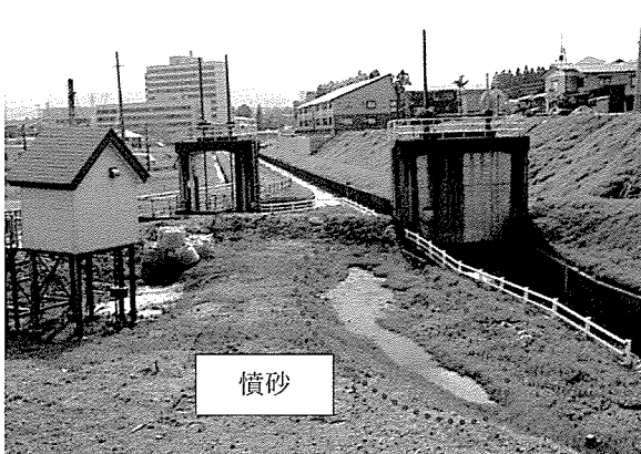
Photo 12 千谷放流工と積砂 Sand gushing in the near Chiya waterway
