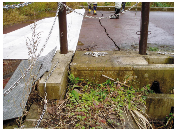
Photo 15 洪水吐取り付け部での段差 Different settlements and cracks at connecting part between the embankment and the spillway at Chofukuji dam
