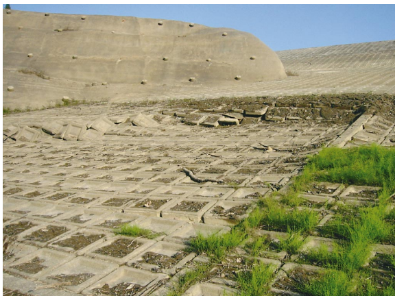
Photo 3 上流斜面の変状 (部分) Damages on the upstream slope (in detail) at Kawanishi dam
