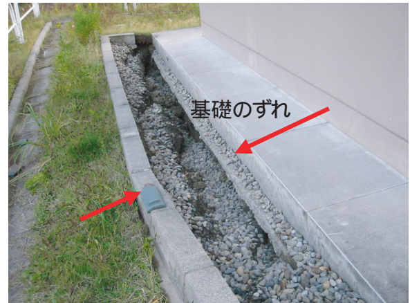
Photo 14 管理棟基礎のずれ Slide of footing of the inspection building at Tsuboyama dam
