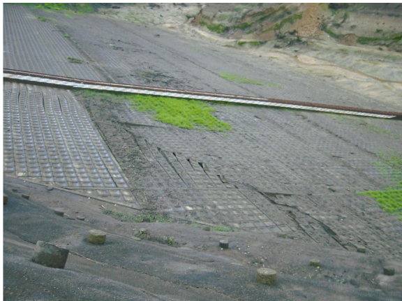
Photo 2 上流斜面の変状 (全景) Damages on the upstream slope (overall view) at Kawanishi dam
