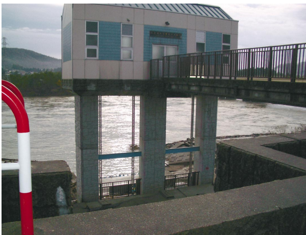
Fig.5 小千谷頭首工取水ゲート門柱 (04.10) Piers of intake gates in Ojiya Headwork
