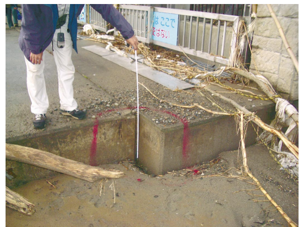
Fig.7 取水ゲート門柱基礎と護岸床との段差 (04.10) A difference level between a pier base and revetment base
