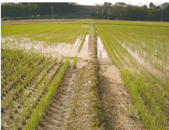
Fig.21 水田畦畔の沈下（04.10） Settlement in the levee of paddy fields
