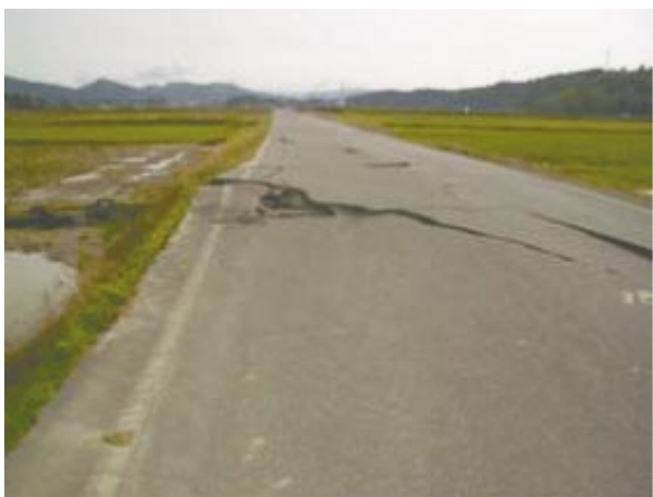
Fig.25 圃場内の農道(幹線)の道路面の損傷(04.10) Cracking on the trunk farm road surface
