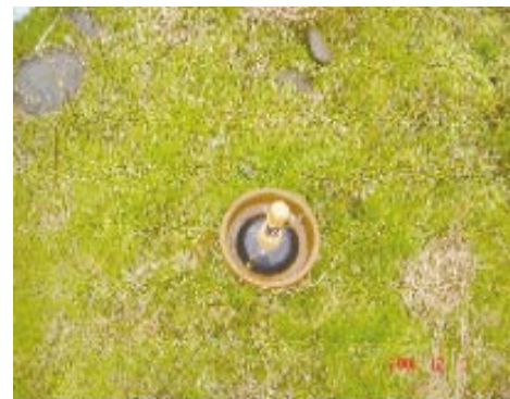
Fig.13 暗渠水閘 Underdrain relief well
