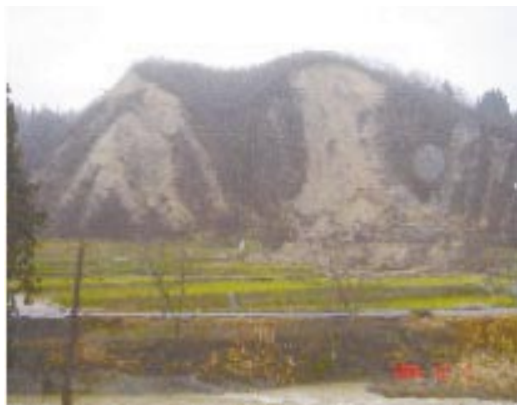
Fig.4 崖崩れに伴う土砂の流入 Inflow of earth and sand by cliff crumble
