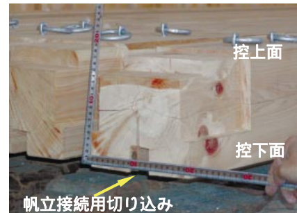
Fig. 7 控の上流端の加工形状 Cutting shape at the upper part of Hikae
