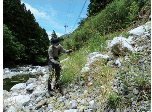
Fig. 22. Riverbank where landslide occurred (FK13).
