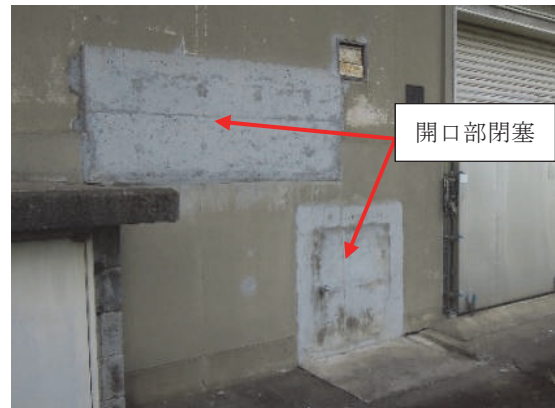
Fig. 4 外壁開口部の閉塞 Removal of the doors and windows on exterior wall
