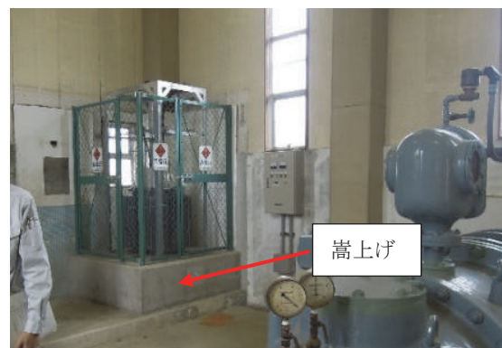
Fig. 5 嵩上げ (電源設備) Raising the platform for the electricity facility
