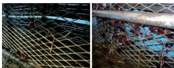
Fig. 27 EMのゴミ付着状況 Condition of trash deposition of expand metal
