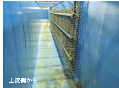
Fig. 9 GC の設置状況 Outline of sheet along side wall
