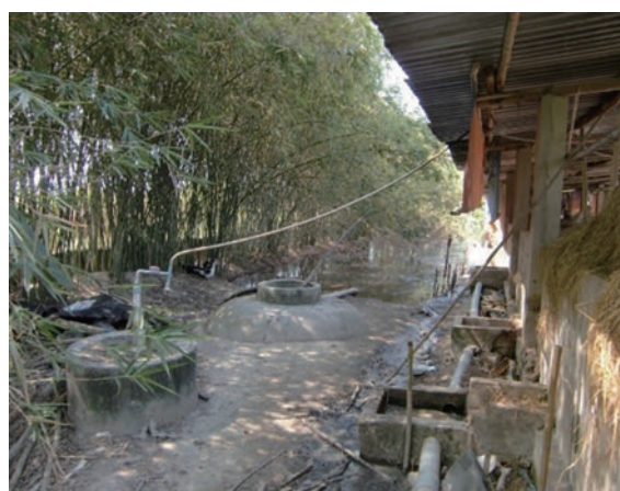
Fig. 7 Biogas digester in a pig farm
